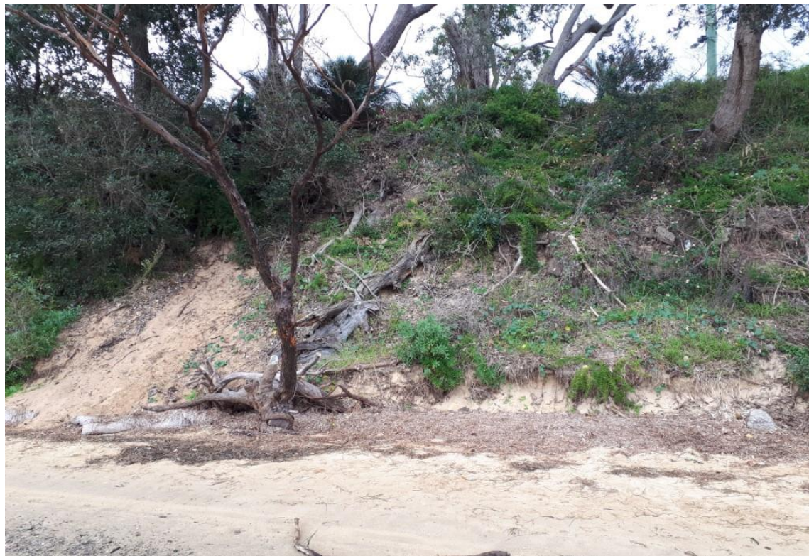
Photo 8. Embankment showing sand slip, dead trees and weedy, patchy vegetation
