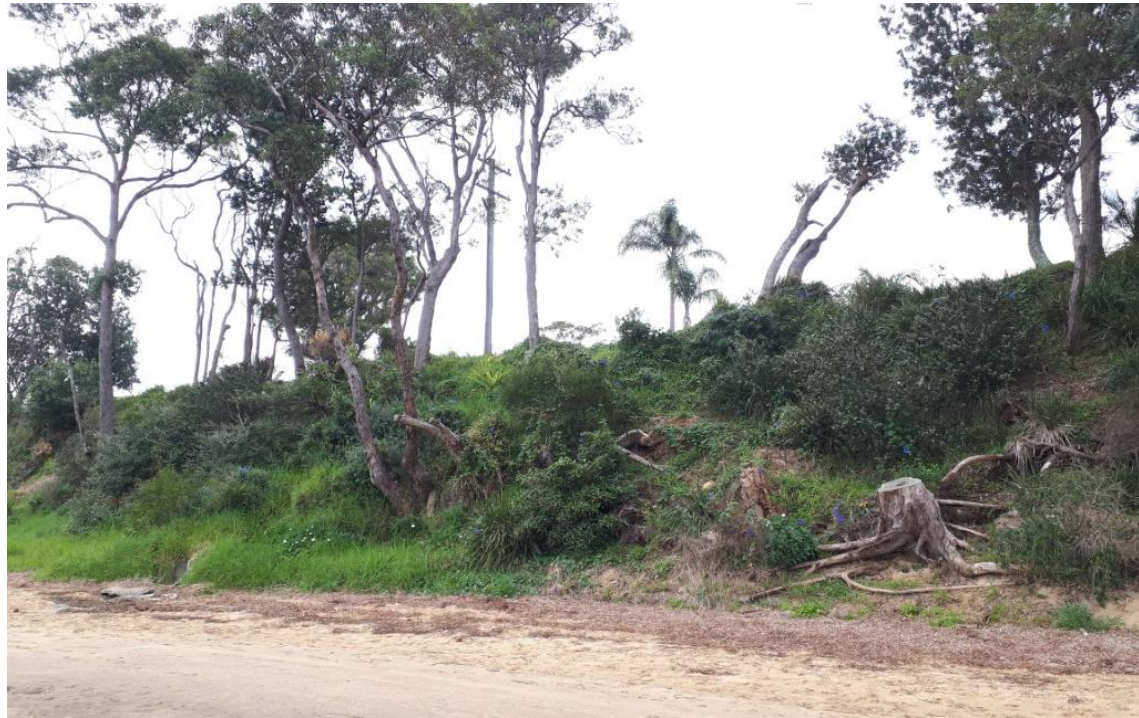
Photo 8. Embankment showing sand slip, dead trees and weedy, patchy vegetation
